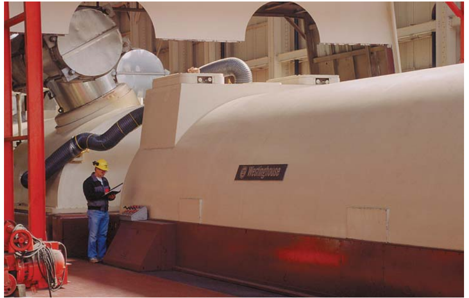
As the unit came off line, the generator housing began to collect condensation. The system was modified to protect the generator by pulling a small amount of dry air from the low pressure turbine through the flexible hose shown here.
