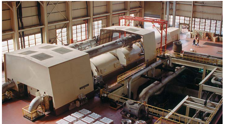
Munters technical support personnel worked in partnership with the plant staff to plan and execute the dry air system. Full support through the end of the outage was essential, because equipment had to be relocated and readjusted as construction proceeded through different parts of the unit.
