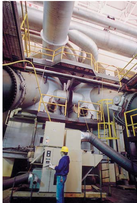
A Munters dehumidifier injects dry air into the hotwell of the condenser. From there, the air flows back through the water/steam side, eventually returning to the dehumidifier via the condensate pumps.
